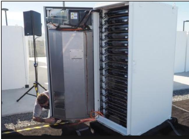
Figure 6: Solid state battery module
